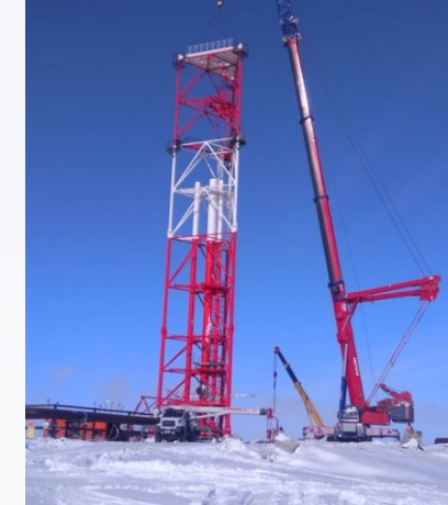
Combined flare unit with forced air supply
