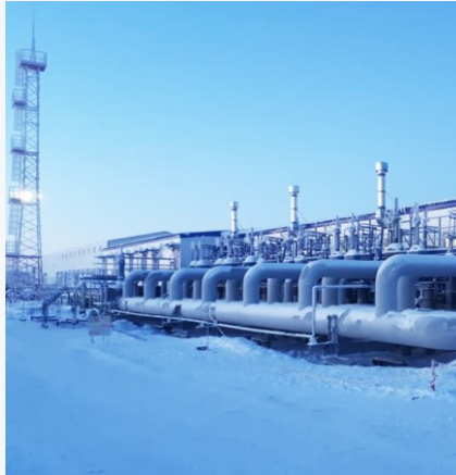
Modular water pump station
